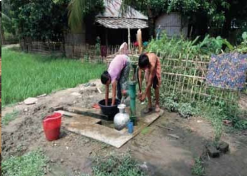
Shallow tube well installed under the project intervention
